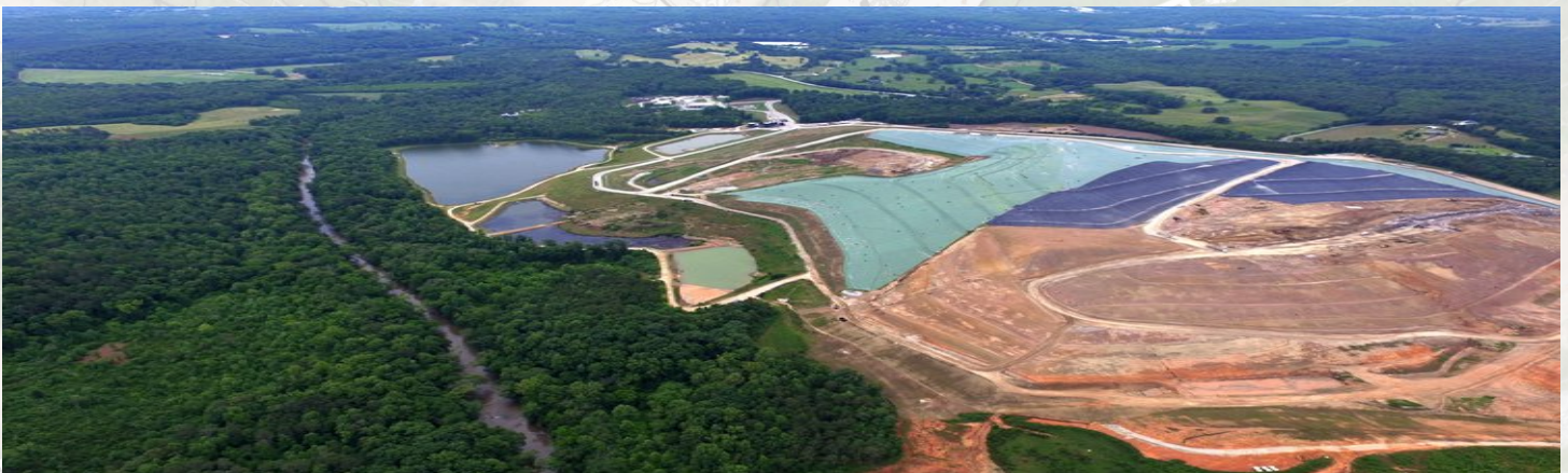
Eagle Point Landfill, Ball Ground, Georgia. We know what it takes to make a RNG facility perform well.
